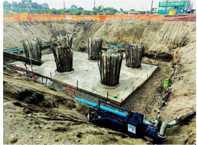
Malolos-Clark Railway Project (2023)
