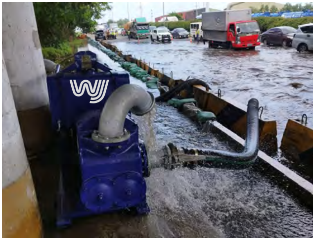
Emergency Flood Control at NLEX in San Simon (2023)
