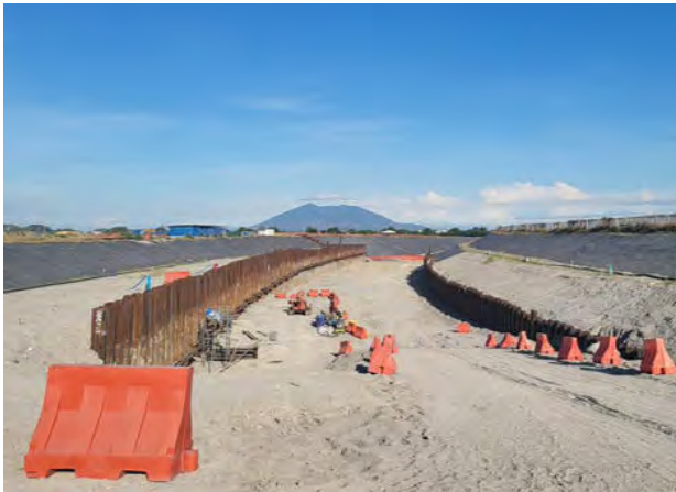
Malolos-Clark Railway Project (2022)
