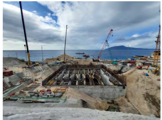
Over Pumping in Combined Cycle Power Plant (2023)
