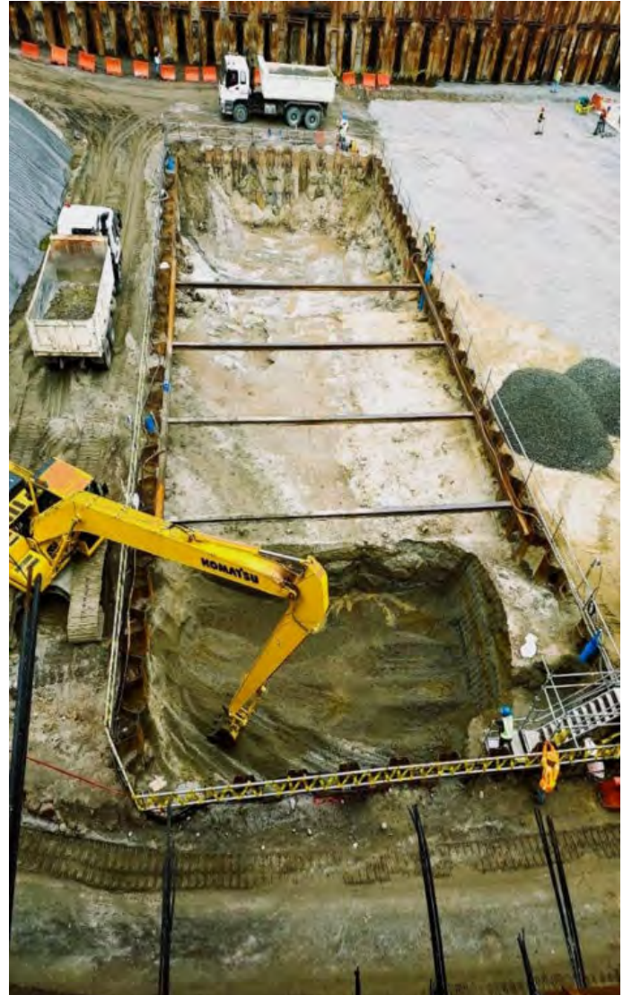
Malolos-Clark Railway Project (2023)
