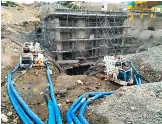
Over Pumping Project in Batangas (2022)
