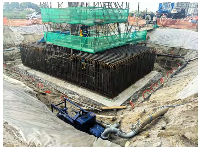
Malolos-Clark Railway Project (2023)
