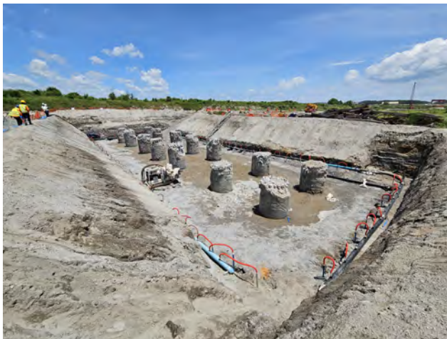
Malolos-Clark Railway Project (2022)
