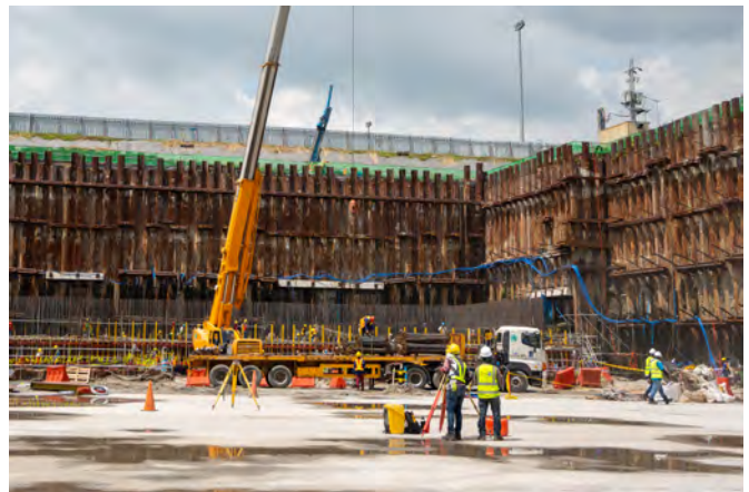
Malolos-Clark Railway Project (2023)
